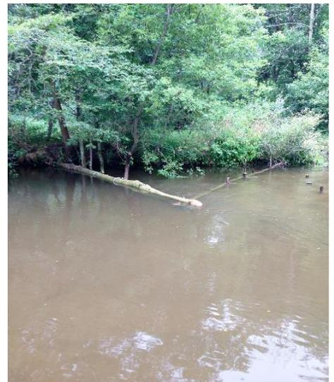
A triangular crib structure was built at the downstream end of the wall to deflect the current away from the wall towards the opposite bank and to create some overhead cover. All along the wall the base log will provide cover from above and the current will scour out a deep run at the base of the wall. Upstream of the wall another current deflector will be built on the opposite bank to divert the current over against the wall.
